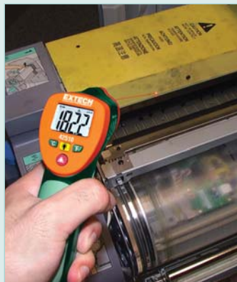
Electrical Troubleshooting for hot spot detection
